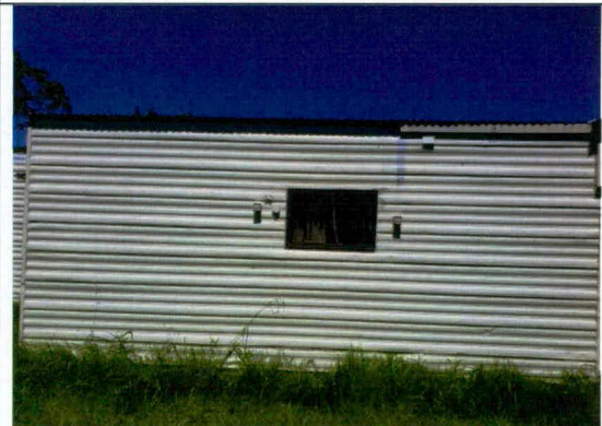
Photo 7 seal the roof and wall junction to fill gaps greater than 3mm.: This can be done using a mesh of perforated sheet with a maximum aperture of 2mm and made of corrosion -resistant steel, bronze, or aluminum or mineral wool or some other non-combustible material.
