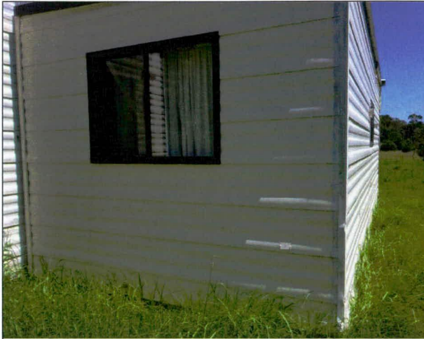
Photo 4: openable windows will require metal screens that comply with AS 3959-2009 or have a mesh with a maximum aperture of 2mm and made of corrosion resistant steel, bronze, or aluminum. There must be NO gaps greater than 3mm. The frame supporting the mesh should be metal, and, or a timber specified in AS 3959-2009
