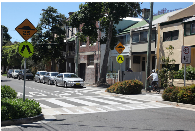
Raised pedestrian crossing on George Street, Redfern. Image - (ASPECT Studios)
