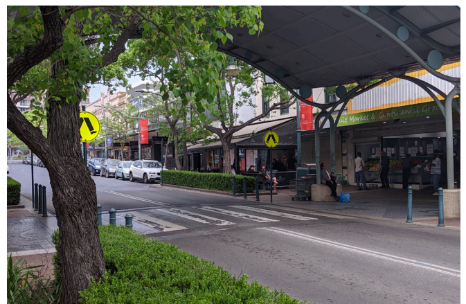
Flush pedestrian crossing on Macquarie Street, Liverpool. Image - (ASPECT Studios)
