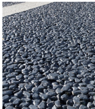
Permeable Asphalt Image - (construction climate challenge)
