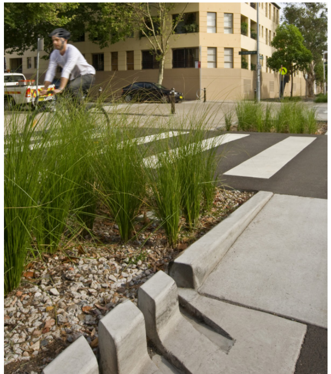
Kerb cuts for passive irrigation on Bourke Street, Surry Hills. Image - Bourke Street Cycleway, City of Sydney (Simon Wood)
