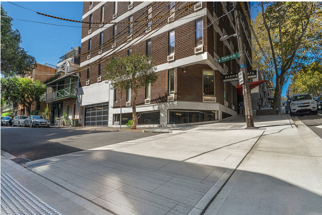
A continuous footpath allows for safer pedestrian travel. Image - Foveaux Street, City of Sydney
