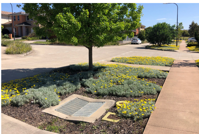
Planted swale in Eckersley Way, Moorebank. Image - (ASPECT Studios)
