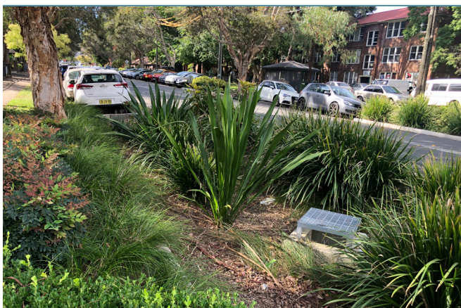
A densely planted raingarden along a street in Sydney. Image - (ASPECT Studios)
