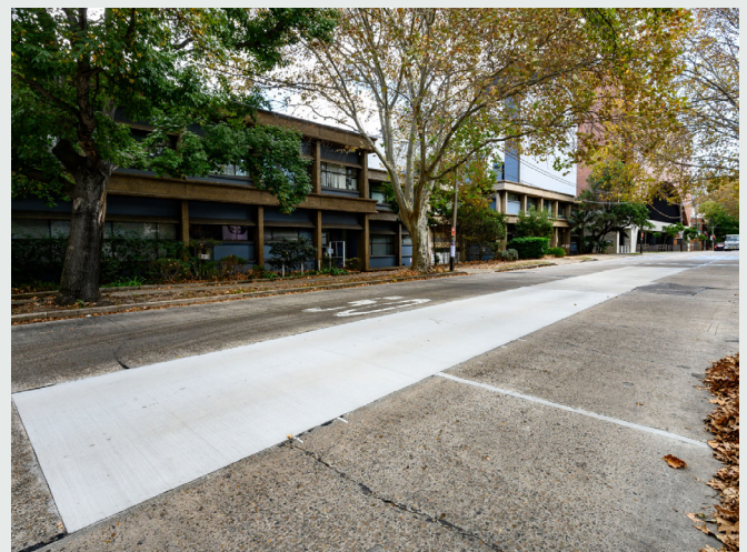
'Green concrete' on Wyndham Street, Alexandria Image - (City of Sydney)
