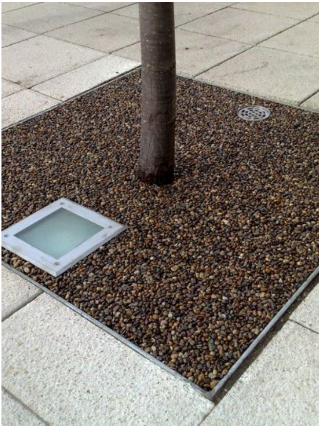
Tree pit Terrabond Image - (Resin Drives)
