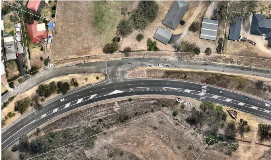
Argyle St, Picton (Jarvisfield Rd)
