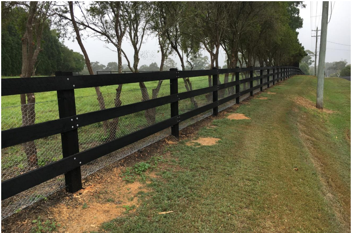
Figure 4.6.1 Example of 1200mm high timber post and rail fence with chicken wire mesh
