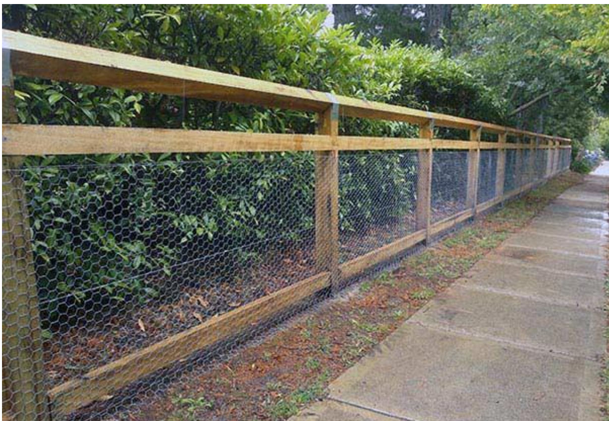
Figure 4.6.2 Example of 1200mm high timber post and rail fence with chicken wire mesh
