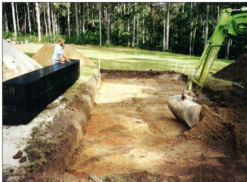
Figure 8.3 Excavation/preparation of base of mound (Figures 8.3-8.7 Ecomax, 2001)
