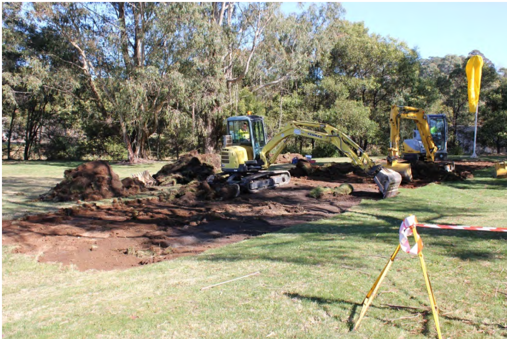
Figure 9.2 Excavation/preparation of base of mound
