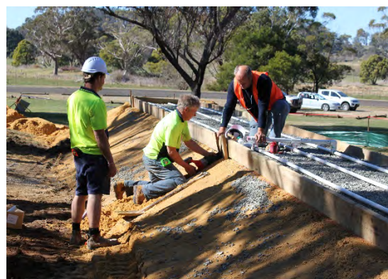
Figure 9.4 Constructing the manifold
