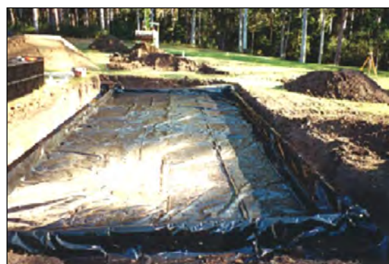
Figure 8.5 Lining with an impervious liner
