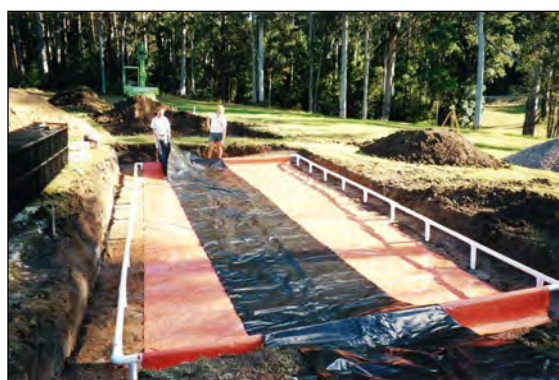
Figure 8.4 Construction membrane
