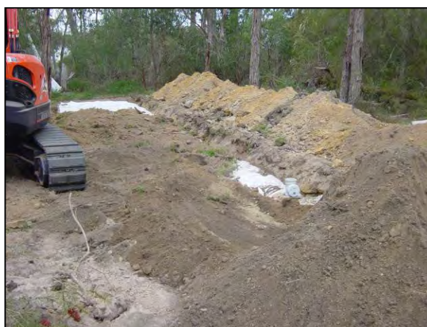
Figure 10.20 Backfilling and the inspection ports
