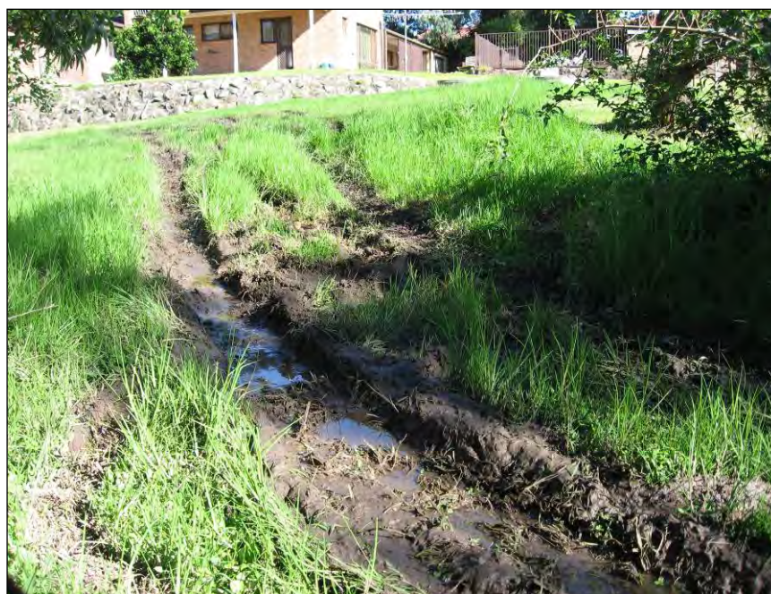
Figure 10.7 A failing trench due to vehicular activity
