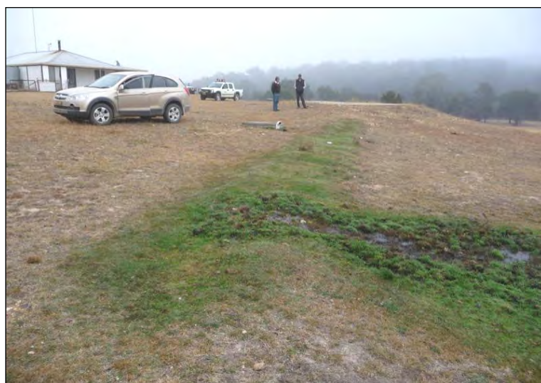
Figure 10.10 Failing trench
