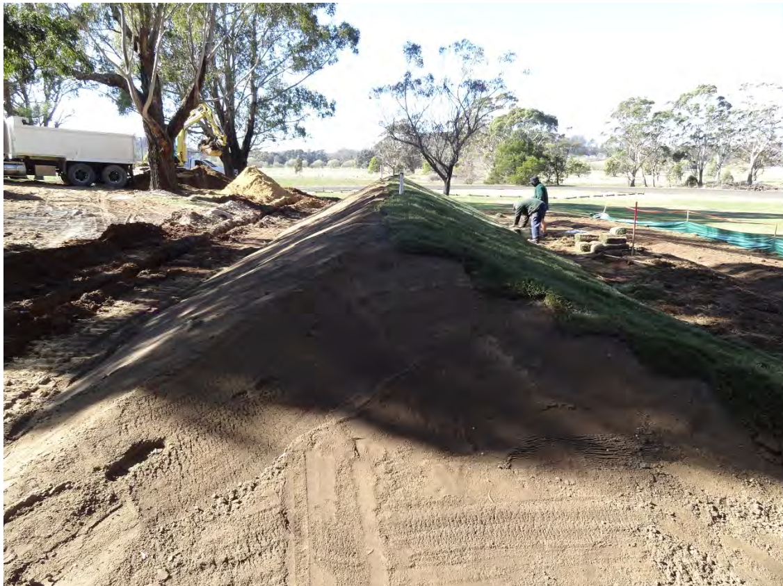
Figure 9.7 Turfing the mound
