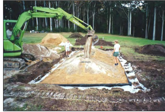
Figure 8.7 Final shaping of cell mound
