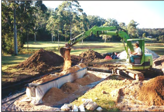
Figure 8.6 Backfilling with amended soil
