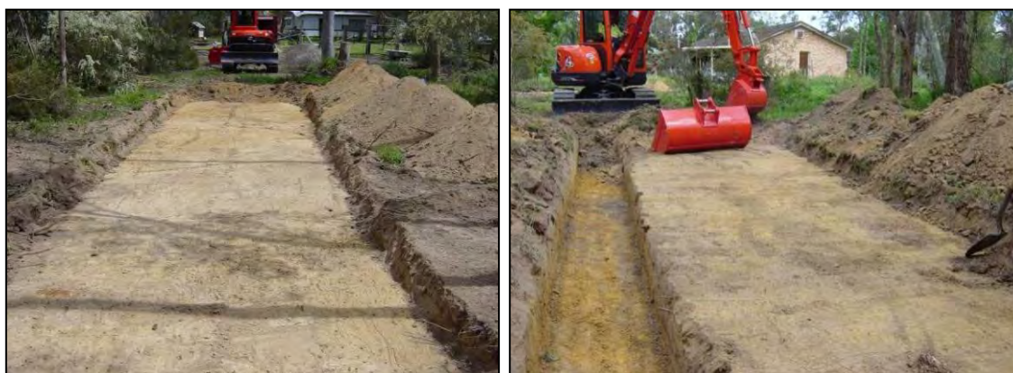
Figure 10.14 and 10.15 Excavation of the bed of the “Wick” trench
