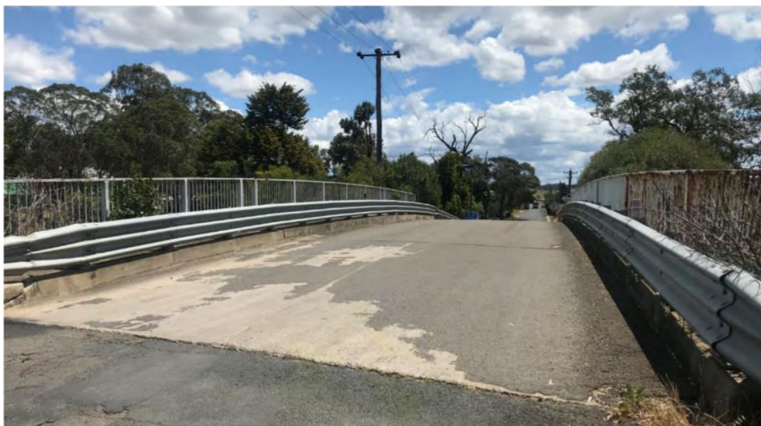
Photograph 1: Existing Station Street Bridge
