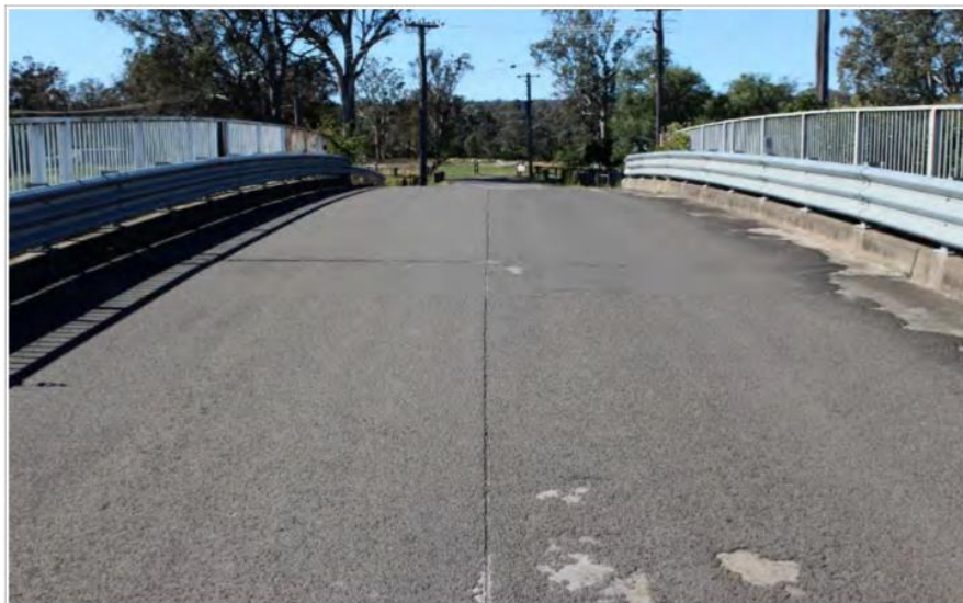
Plate 2 - Surface view of deck
