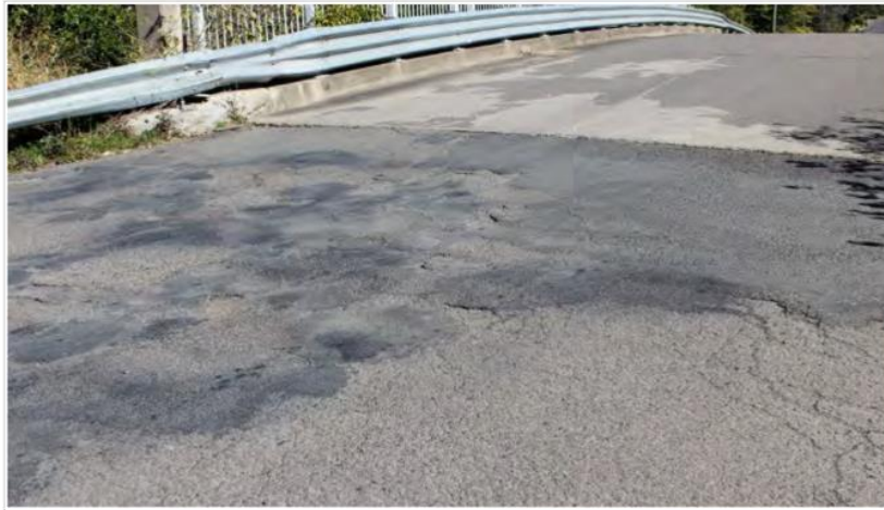
Plate 3 - Approach to Abutment B
