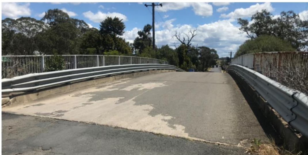
Photograph 1: Existing Station Street Bridge
