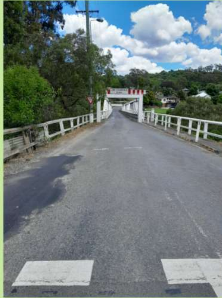
Photo 2: Approximate driver view at westbound hold position.
