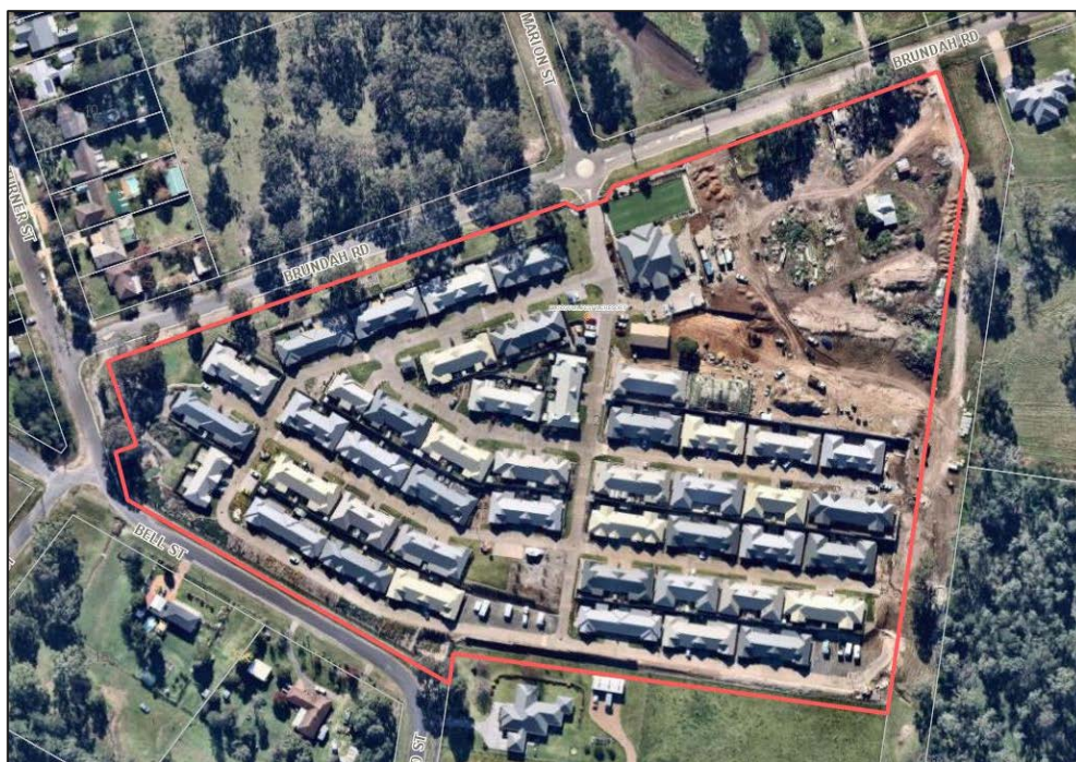
Figure 1 Aerial Imagery (Source - NearMap 28 May 2017)
