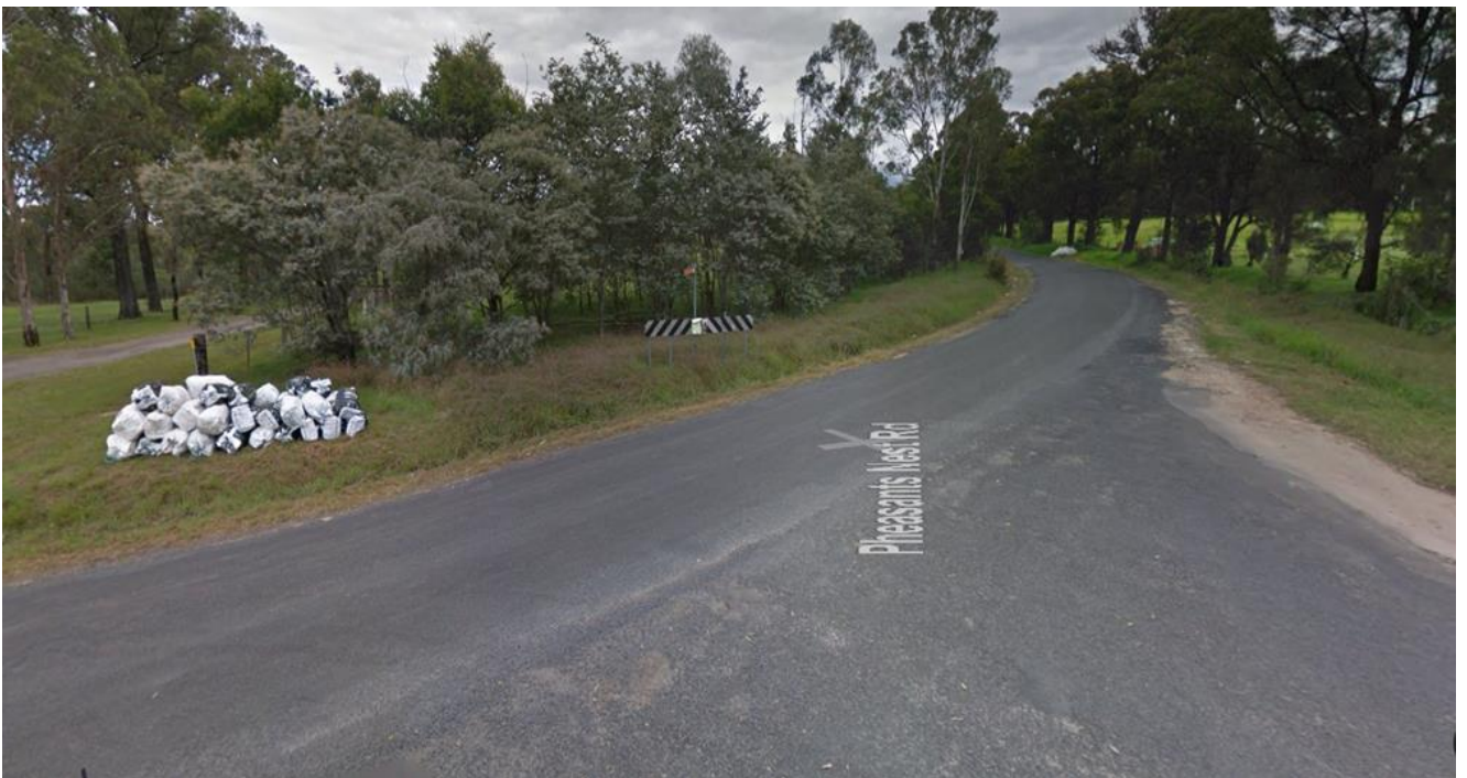
Lyrebird Rd at Pheasants Nest Rd, - Existing holding lines and insufficient safe sight distance
