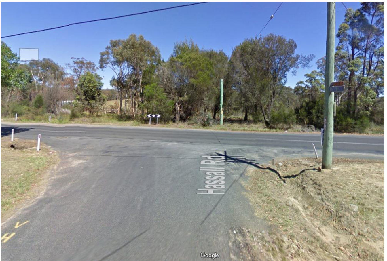
Hassall Rd at East Parade, Buxton - Reported incidents of traffic not giving way especially during school peak hours and insufficient safe sight distance
