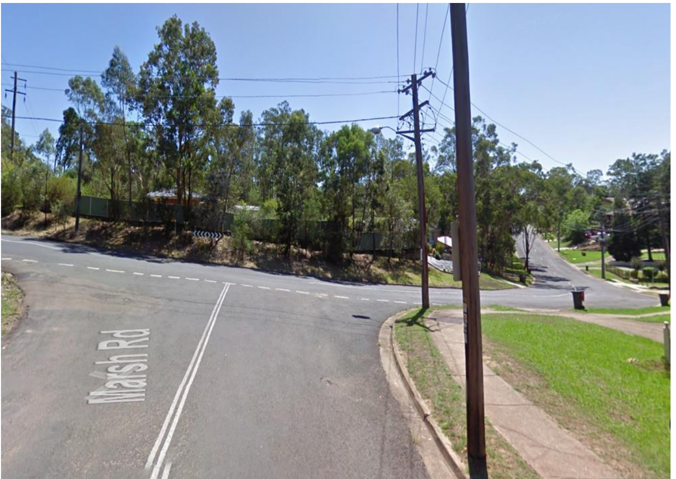
Marsh Rd at Warradale Rd, Silverdale – Existing holding lines and insufficient safe sight distance
