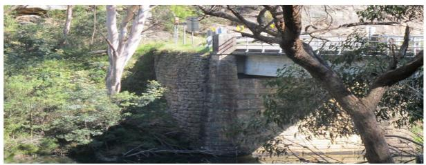
Photo 1 – Extracted from Coffey's Geotechnical Investigation and Concept Design Report, Aug 2016 - View of the western bridge abutment and dry packed stone wall supporting the road formation on the southern side of the road approach to the bridge, before the damage (Picture taken in September 2011).
