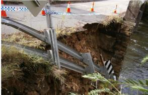
Photos 2 & 3— Extracted from Coffey's Geotechnical Investigation and Concept Design Report, Aug 2016 - View of the failed bridge and retaining wall observed on 6 June 2017.
