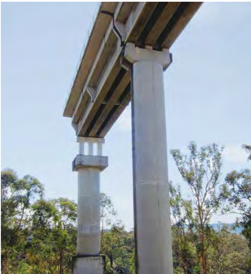
View North across unfinished railway bridge.
