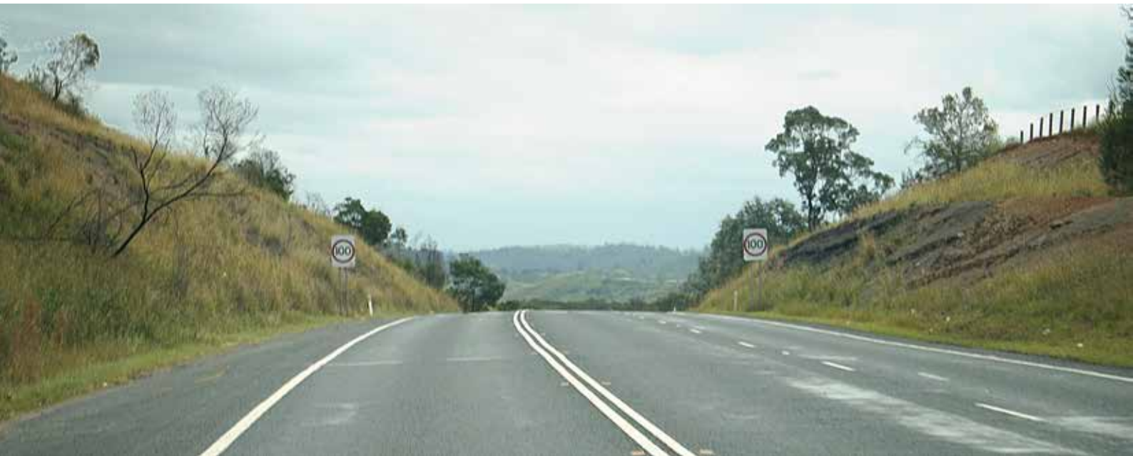
View of Picton Road Cutting Looking West
