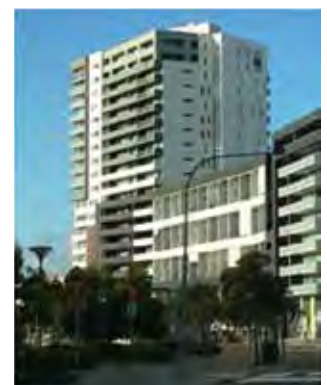
Wollri Creek (Discovery Point): max 60m (20 stories) and building specific GFAs to 41,000sqm;
