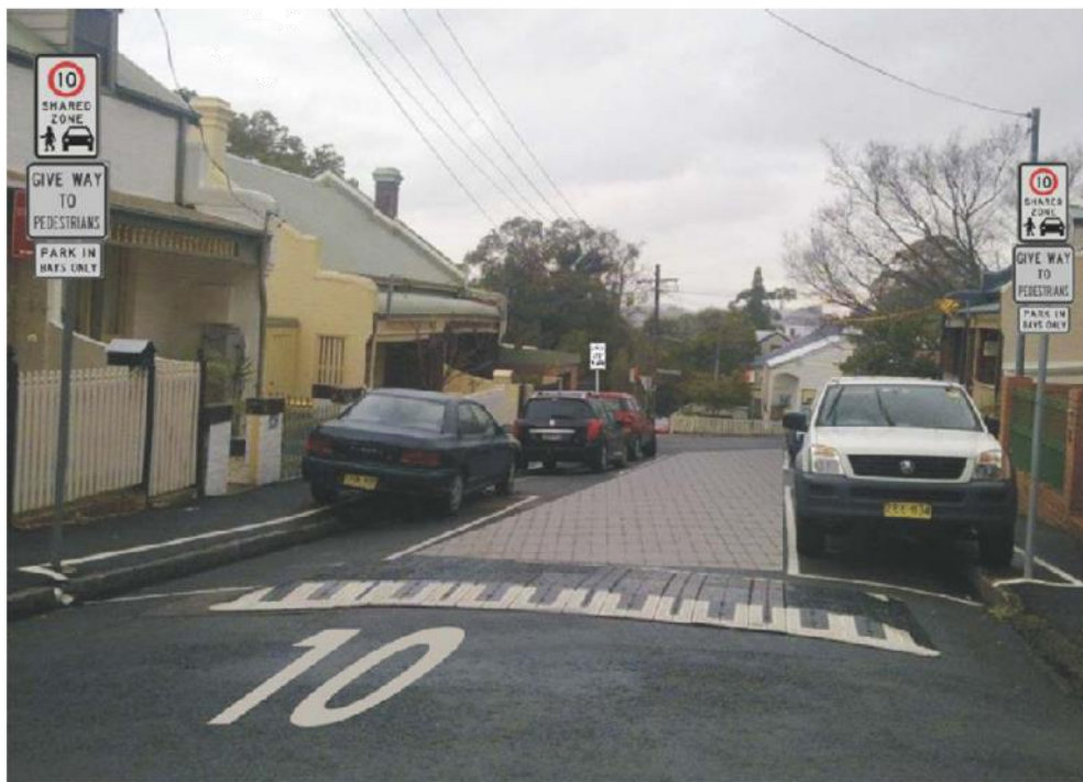
Figure 2. Photo and diagram of a Category 2 shared zone showing treatments, traffic calming, parking provision, and typical layout. 'Give Way' to Pedestrian' pavement marking is optional.
