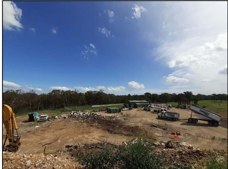
Figure 9: The Bargo Waste Management Centre's landfill is nearing the end of its operating life.
