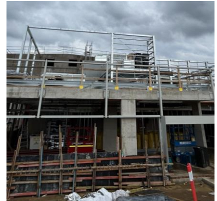
Back-Fill OSD Tank, Mechanical Hobs & Plinths, Stair #2, Completed BOH Structural Steel
