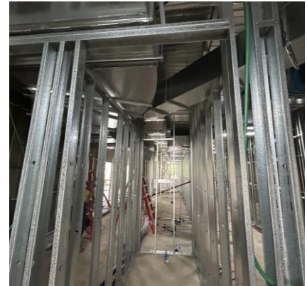
Main Theatre, Wall Frames and Services Rough-in, Insulation Install
