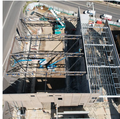
Precast Panels & Structural Steel
