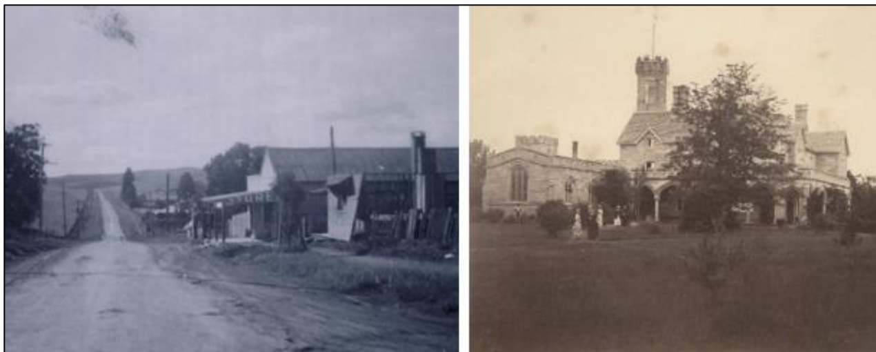
Figure 2-1 Historic photos of Railway Heritage Cottage (left) and St Marys Towers (right) (Source: https://www.joseflebovicgallery.com/pages/books/CL181-59/nepean-towers-douglas-park-nsw )
