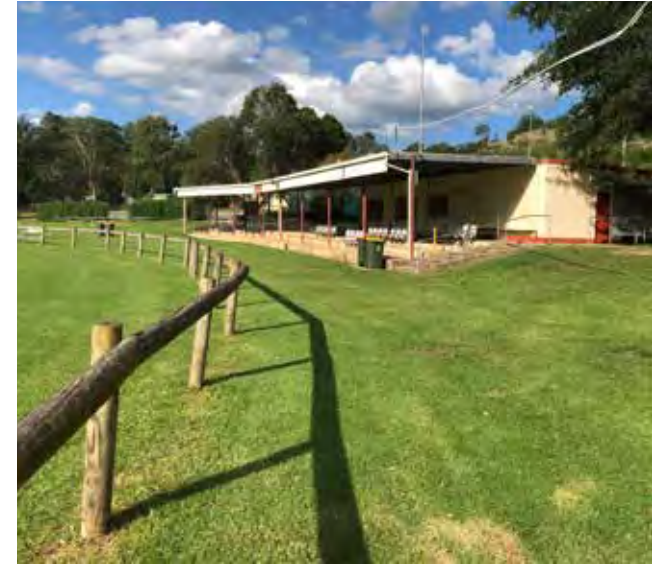
Hume Oval amenities building and grandstand seating
