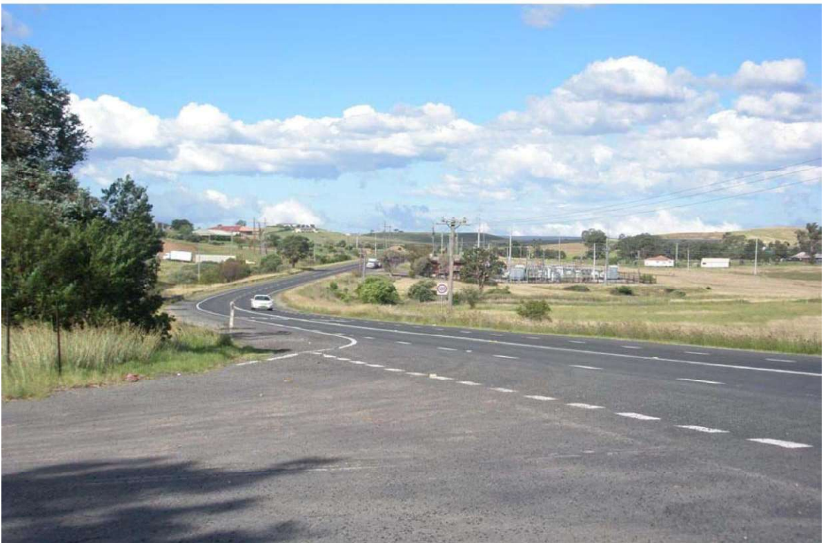
PHOTO B VIEW FROM THE SITE ACCESS TO THE EAST ALONG PICTON ROAD SHOWING THE WIDENED WESTBOUND CARRIAGEWAY OF PICTON ROAD AT THE SITE ACCESS TO PROVIDE A PASSING LANE FOR WESTBOUND TRAFFIC IF VEHICLES ARE WAITING TO MAKE A RIGHT-TURN INTO THE SITE ACCESS.
