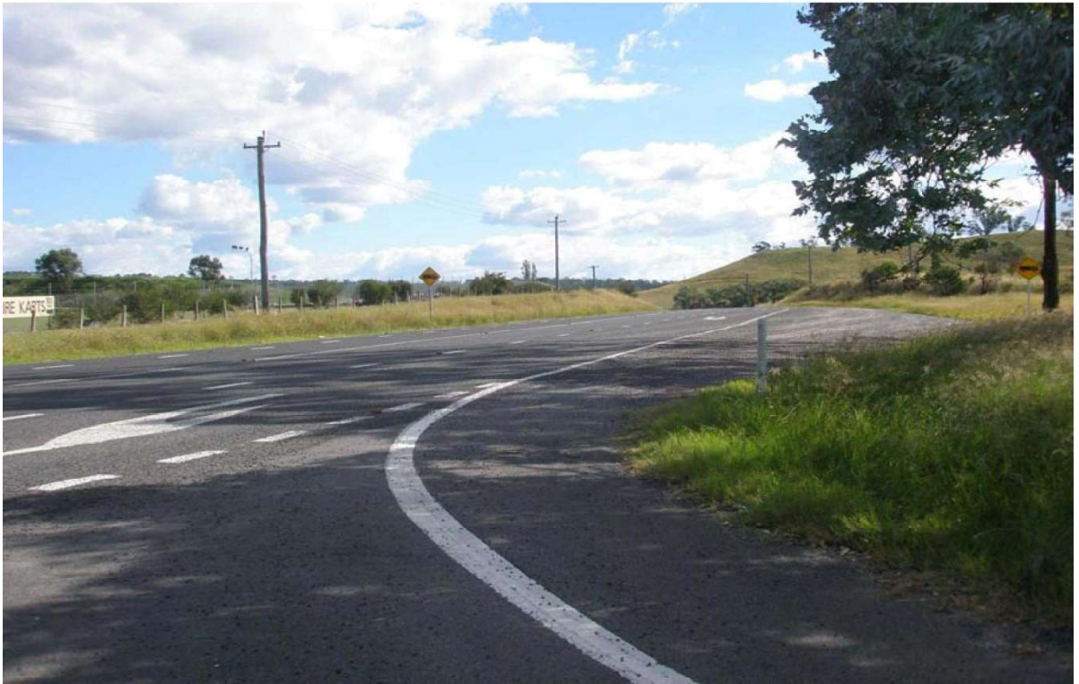
PHOTO A VIEW FROM THE SITE ACCESS TO THE WEST ALONG PICTON ROAD SHOWING THE LEFT-TURN SLIP LANE ON THE EASTBOUND CARRIAGEWAY OF PICTON ROAD ON THE APPROACH TO THE SITE ACCESS
