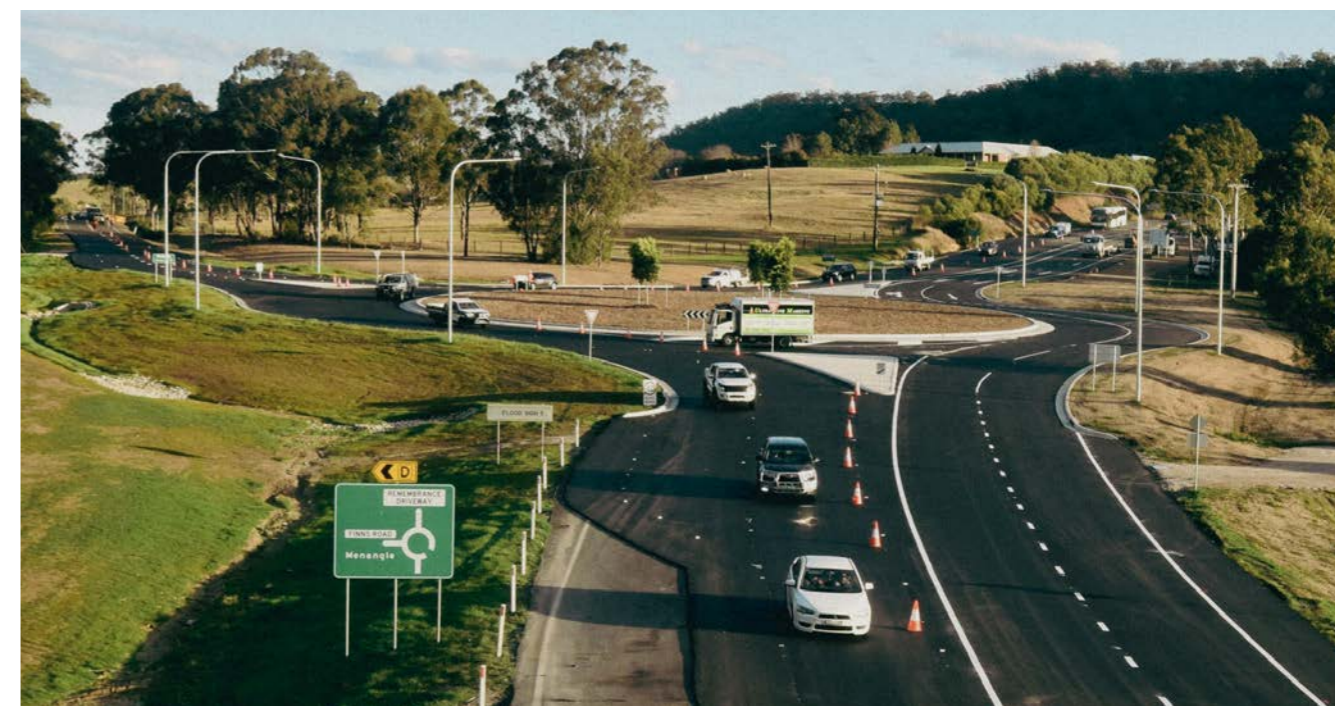
Remembrance Driveway and Finns Road roundabout.
